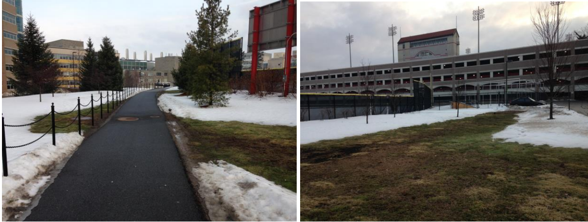
Figures 2-5 and 2-6: Surface snow melt revealing heat loss along steam line (2014)
